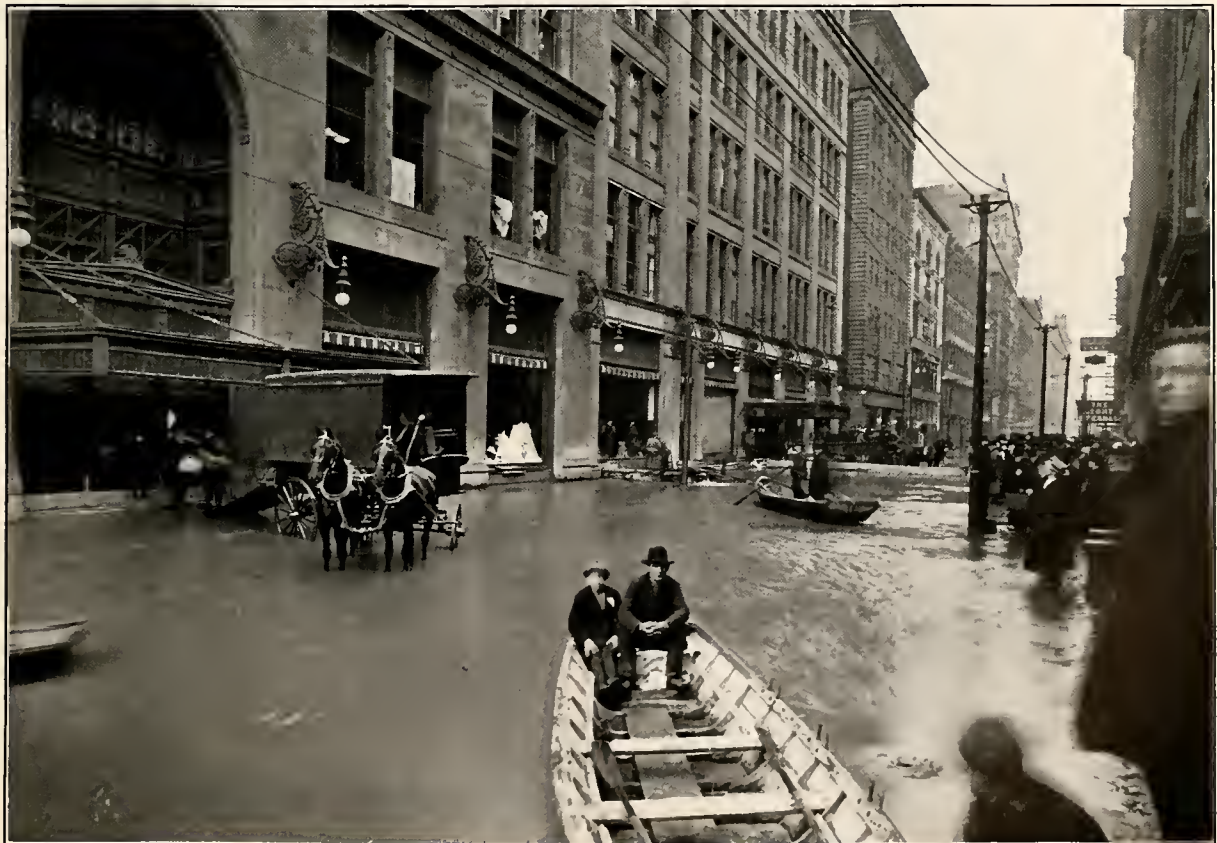
FLOOD OF MARCH 15, 1907. Penn Avenue, looking east from Fifth Street.
